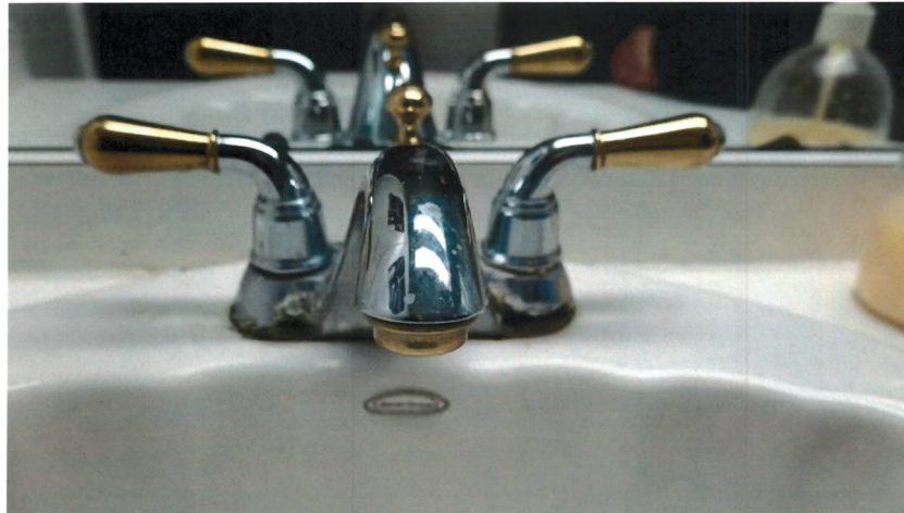
The faucet in Ana Maria Rodriguez's bathroom sink shows signs of corrosion, possibly due to nitrate pollution in Boardman, Ore., Jan. 15, 2023.
